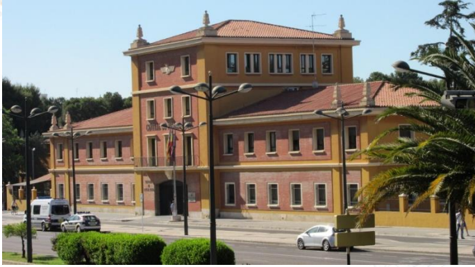
Valencia Local Police Headquarters
